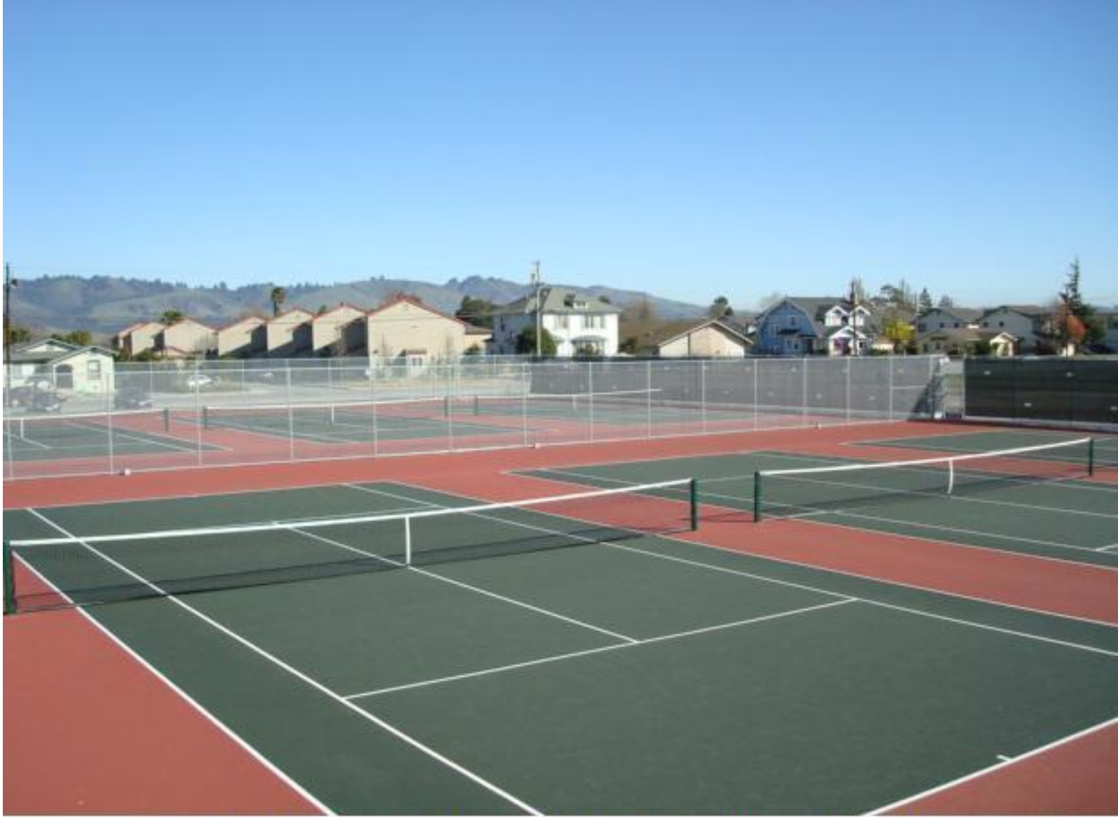
New tennis court facility with six regulation size courts.
