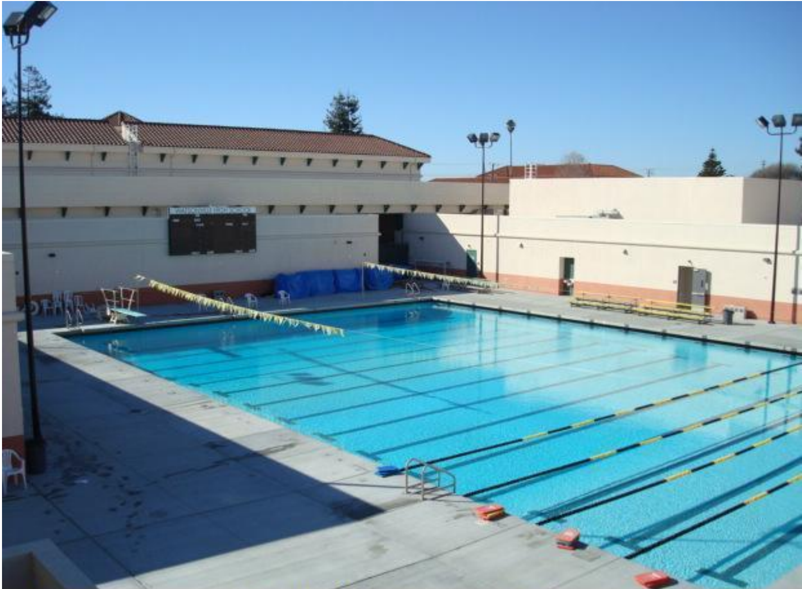
New swimming pool facility (30 meter pool), locker rooms and office.
