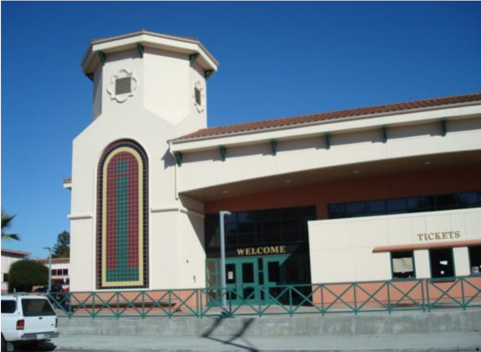
Main entrance and ticket booth to Wildcatz new athletic facility.
